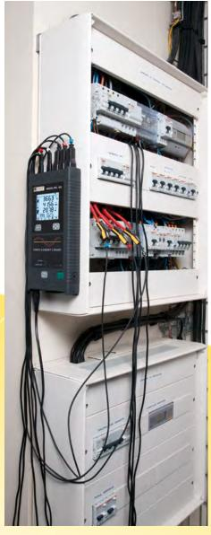
The monitoring by the PEL100 provides the recordings which will be compared with the reference.
